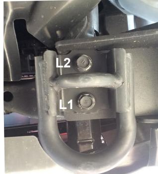
LEFT SIDE SKID PLATE BOLTS
